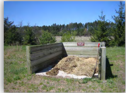
Manure bunker, Sand Dunes State Forest
