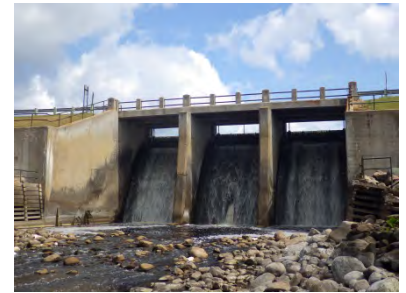
Design and construction of the dam in the 1930s required expertise due to 100' of quicksand that was found at the site.
