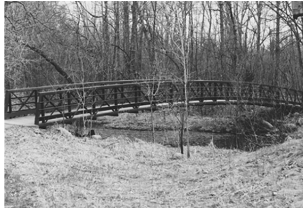
Trail bridge at the site of the original bridge. (circa 1998)
