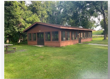
The picnic shelter is enclosed and has electricity. It may be reserved in advanced for events and is open to the public when not in use.
