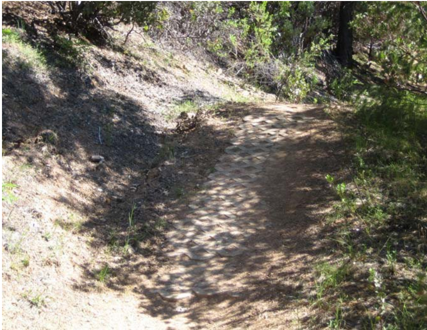
Rolling Dip hardened with paver block (after about 18 years of very heavy use)
