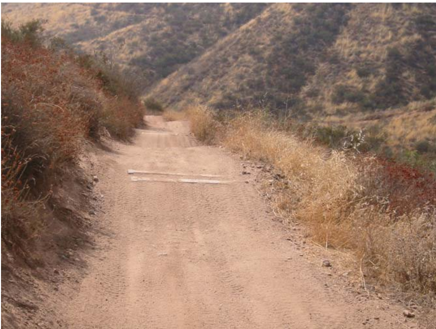
Rolling Dips reinforced with "dog bones"
