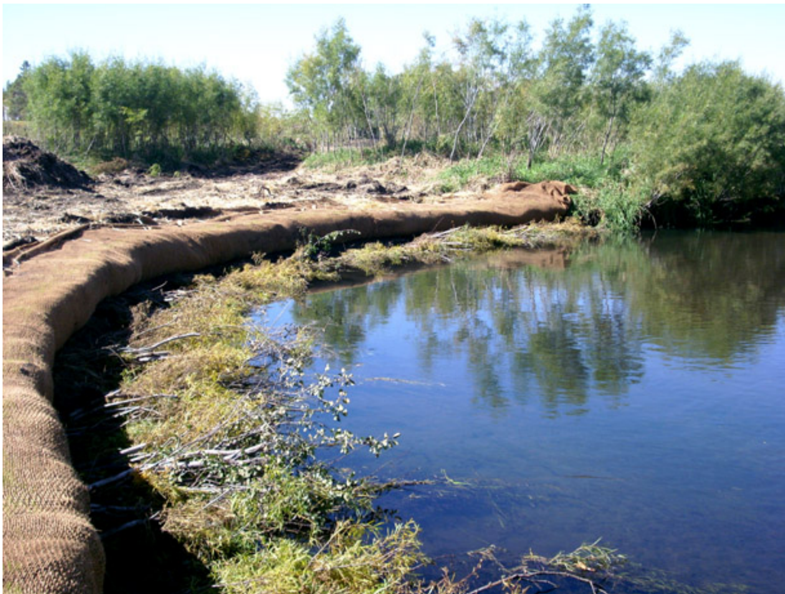
Figure 8. Toewood bank stabilization with encapsulated soil lift.
