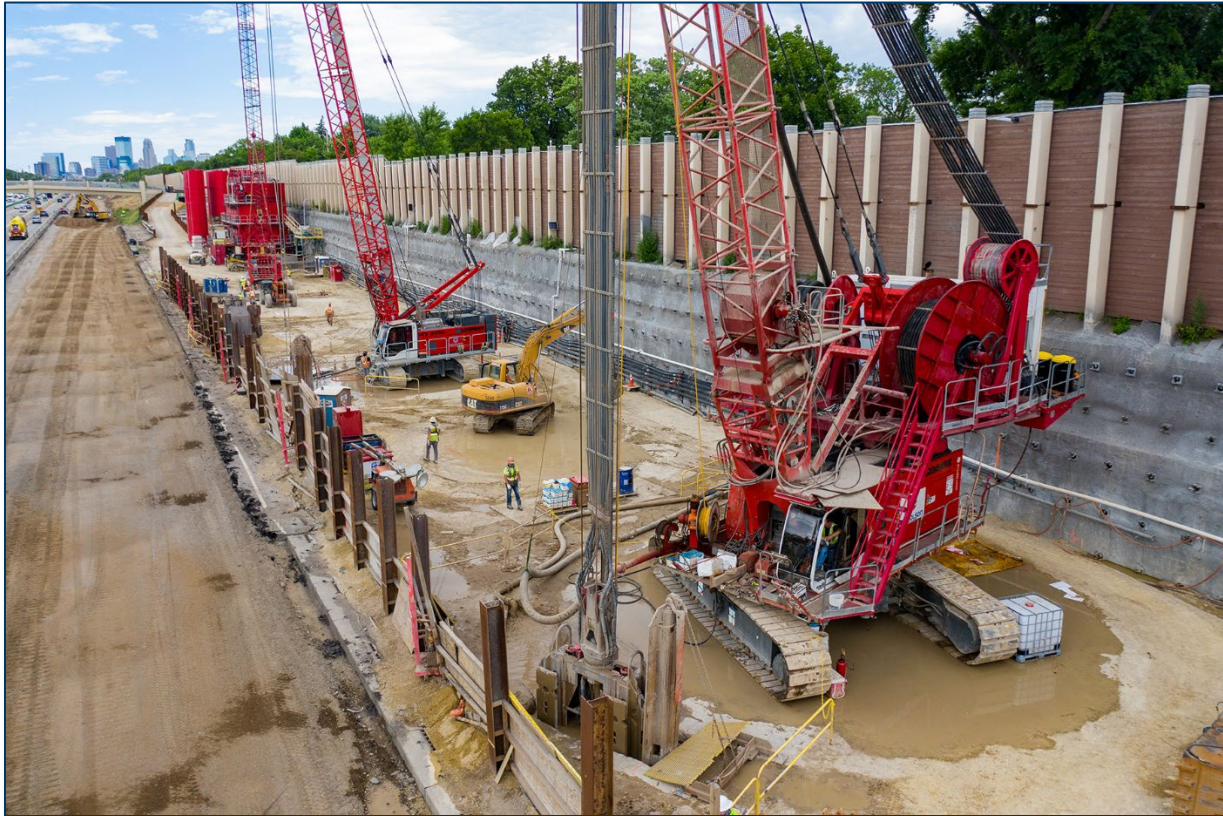
Graphic 6-6 Similar construction methods to the planned cutoff cell were used in Minnesota on I-35 in Minneapolis to prevent the highway from flooding during storm events
