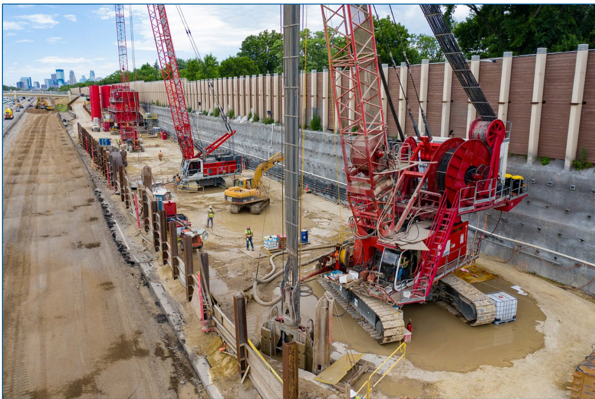
Graphic 6.6 Similar construction methods to the planned cutoff cell were used Minnesota on I-35 in Minneapolis to prevent the highway from flooding during storm events.
