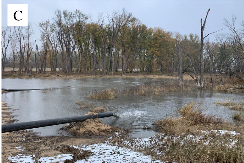
Figure 13. Examples of hydraulic placement with granular containment berms during construction period at the McGregor Lake HREP project in Pool 10 (Wisconsin) from aerial view (A), ground view (B), active hydraulic pumping of dredge material through pipe (C), and hydraulic dredge used for the project (D).
