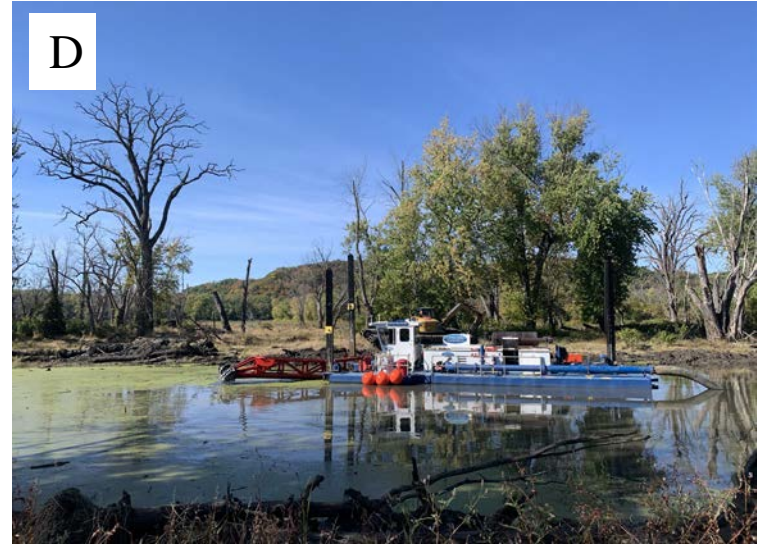
Figure 13. Examples of hydraulic placement with granular containment berms during construction period at the McGregor Lake HREP project in Pool 10 (Wisconsin) from aerial view (A), ground view (B), active hydraulic pumping of dredge material through pipe (C), and hydraulic dredge used for the project (D).
