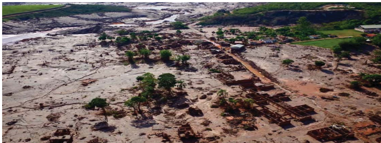
Remains of Bento Rodriguez after failure of Samarco’s Fundao tailings dam.
