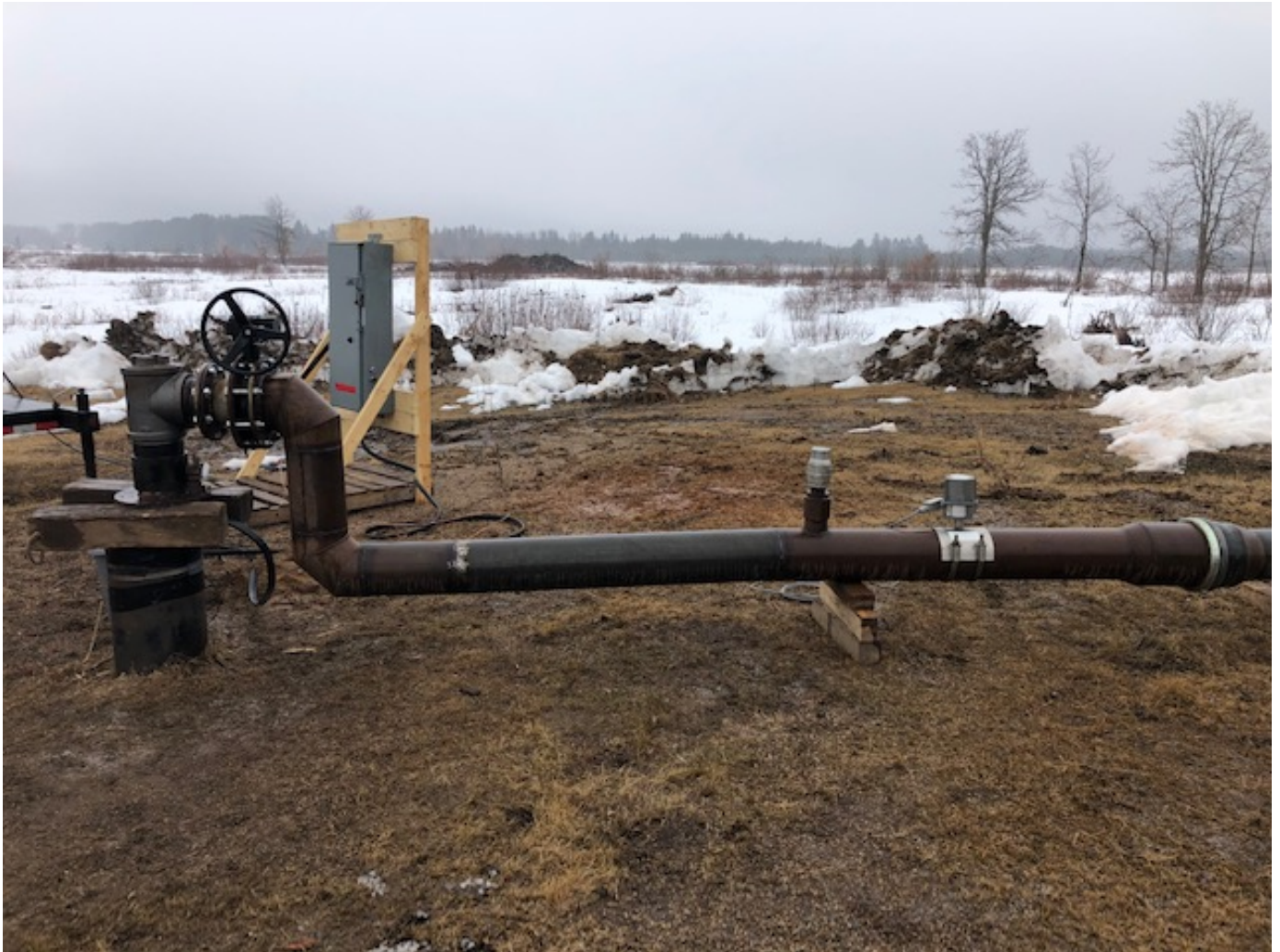
Figure A-1. Production well flow meter set-up
