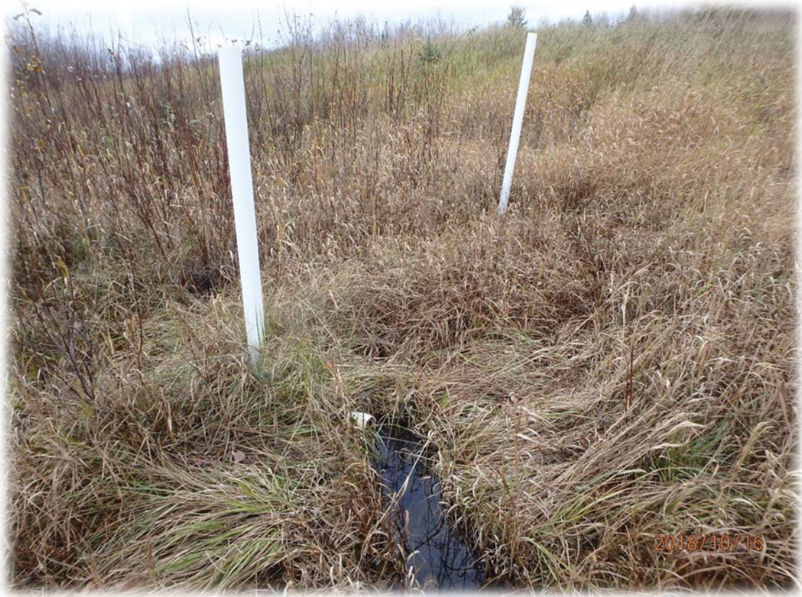
Relief wells at the dam toe
