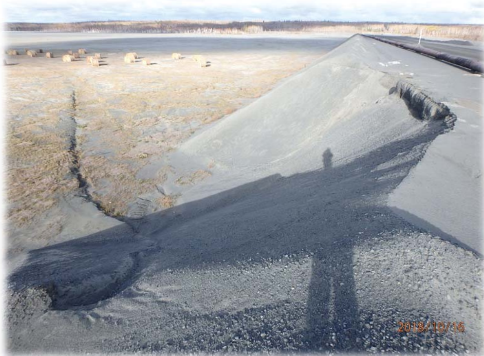
Looking west at some erosion on the filter berm at Dam 2 approximately near station 40+00
