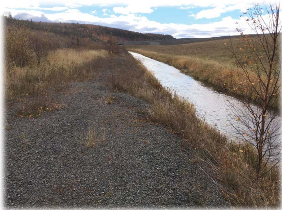
Looking east along seepage collection ditch at Dam 2
