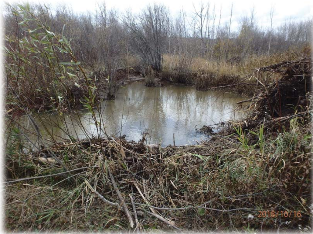
Widened area of drainage ditch off the toe of Dam 2 just upstream of seepage recovery pond 2-3 where beaver dams were removed
