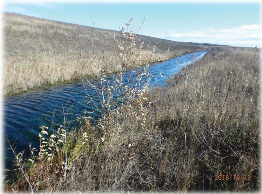
Looking east along seepage recovery ditch with sporadic brush and abundance of algae at Dam 1
