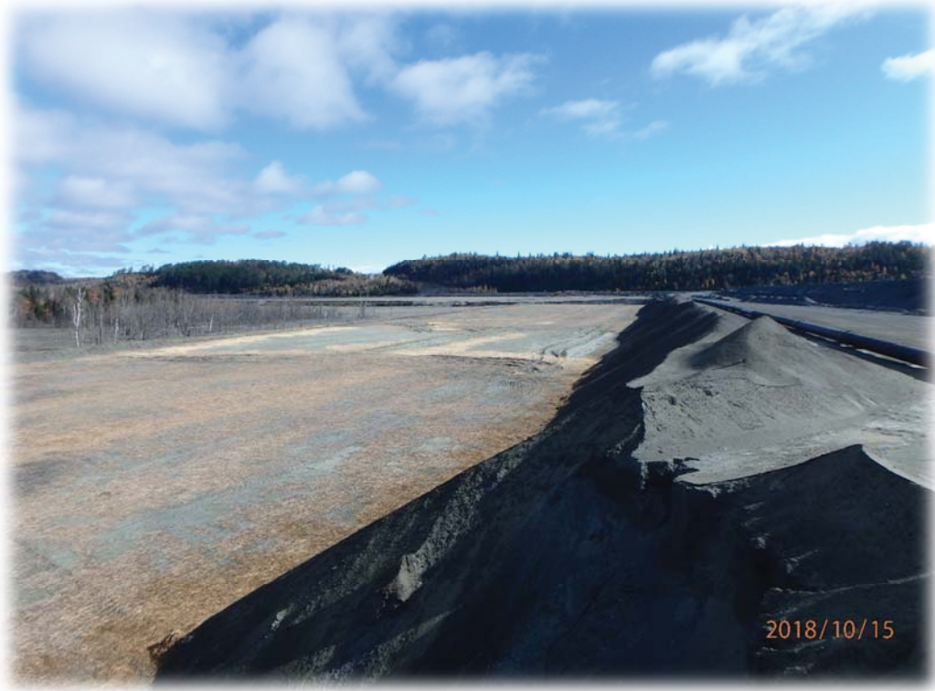
Looking east along filter berm at new super cell beach with original super cell beach in the distance at the eastern end of Dam 1
