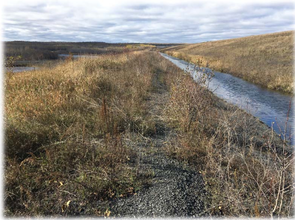
Looking west along seepage recovery ditch from near east weir at Dam 1
