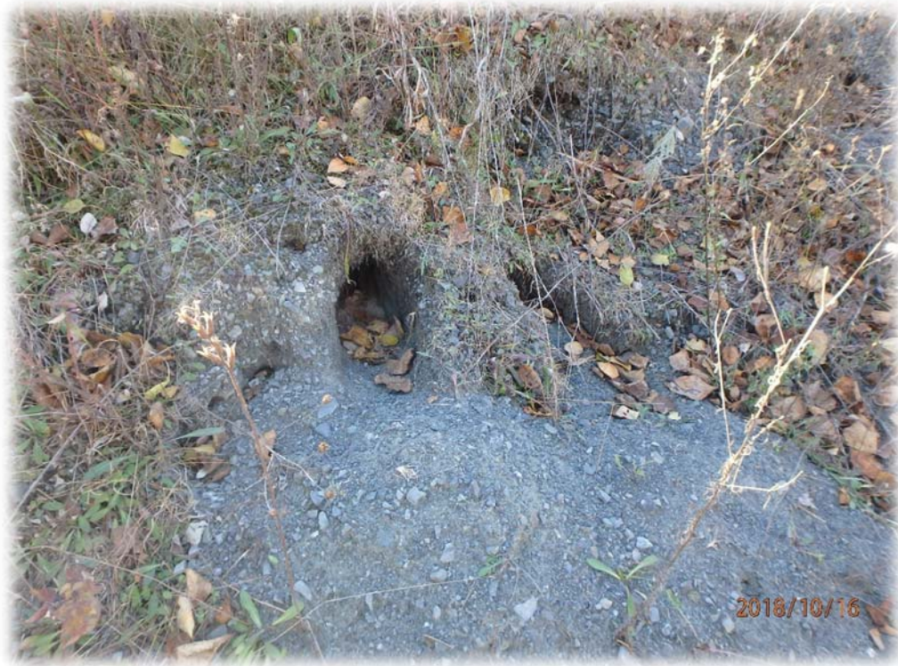
Animal burrows in the filter berm near the weir at the west end of Dam 2
