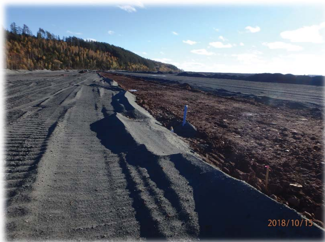
Looking south at recently raised southern portion of Dam 5 near station 14+00
