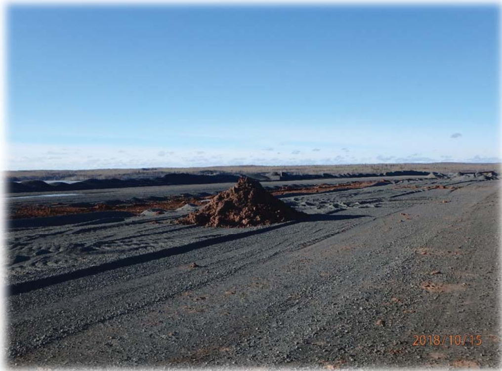
Looking northwest at clay stockpiled on filter material at Dam 5
