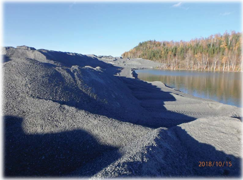
Looking north at buttress extension at the toe of Dam 5
