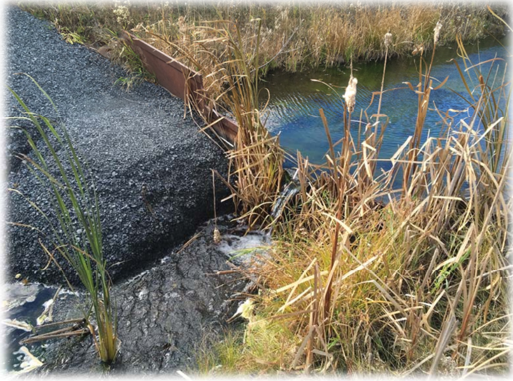
East weir for seepage collection ditch at Dam 2
