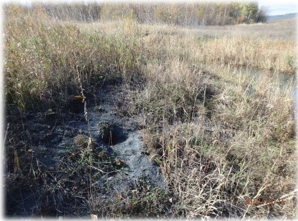
Animal burrows in core at west end of Dam 1, near weir
