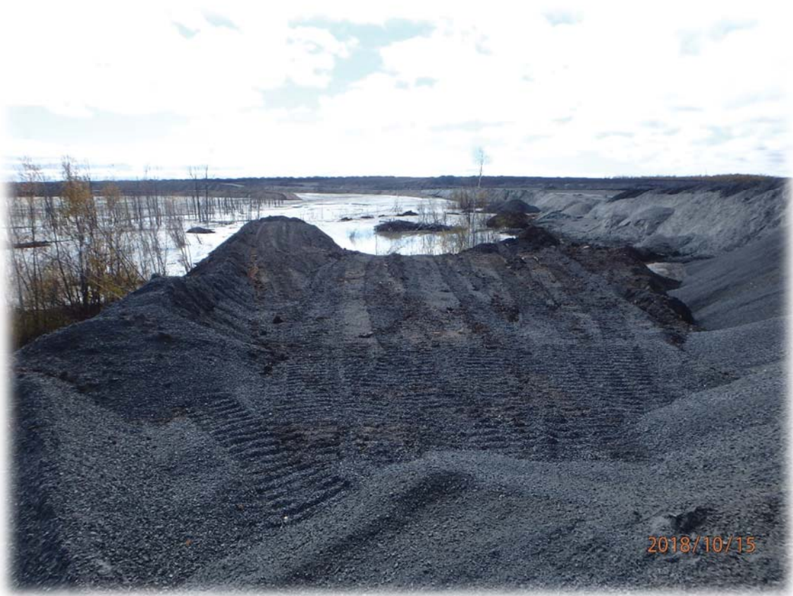
Looking east at filter berm placement at the west end of Dam 1
