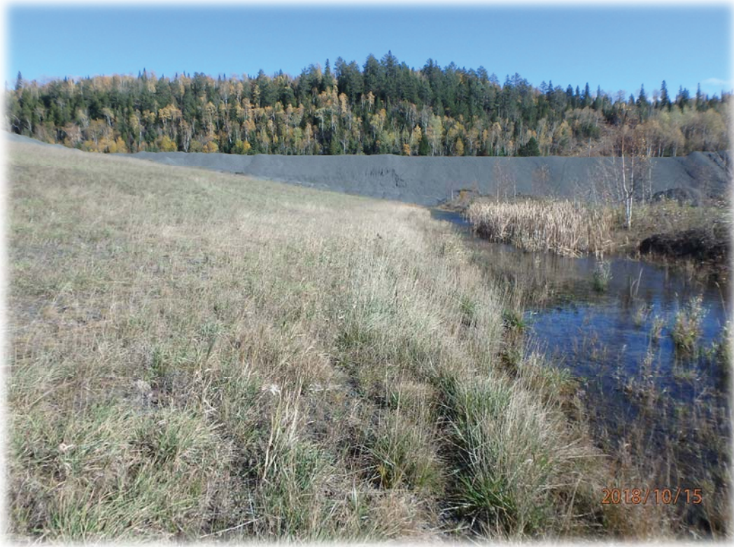
Looking east at seepage collection ditch at the east end of Dam 1
