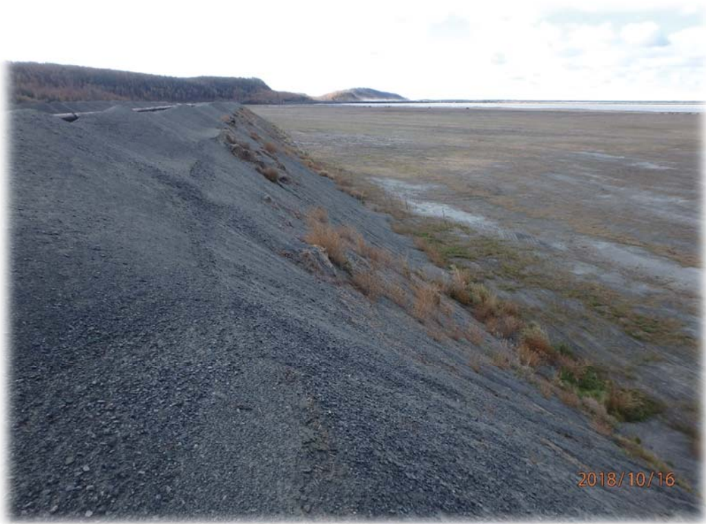
Looking east-southeast at upstream slope of the filter berm of Dam 2
