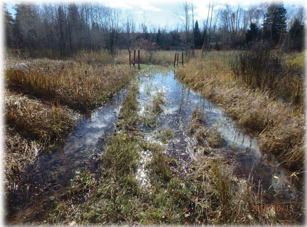
Flooding at west end of the toe of the dam, by monitoring wells
