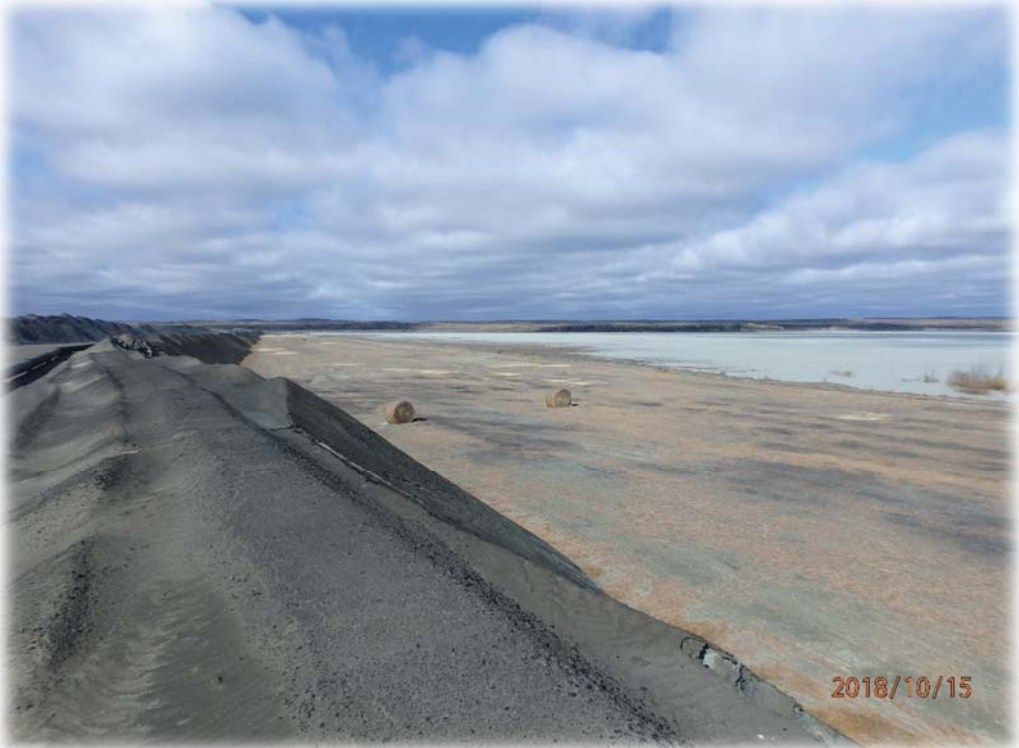
Looking west along the filter berm near intersection of Dam 1 and Dam 1E at new section of mulched super cell beach
