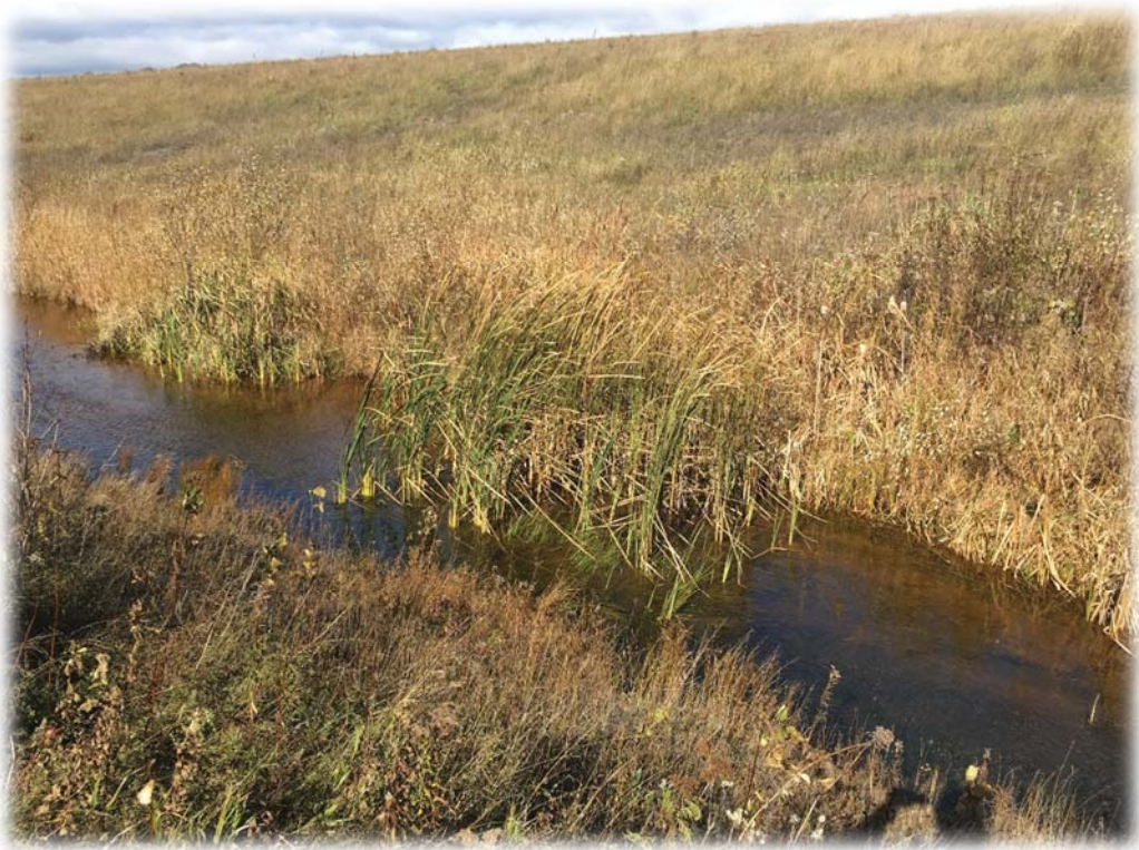
Looking northwest at cattails in seepage recovery ditch near east weir at Dam 1
