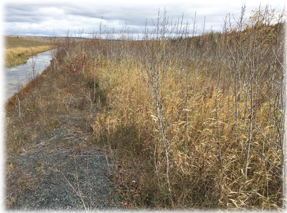
Brush on core near east end of Dam 2
