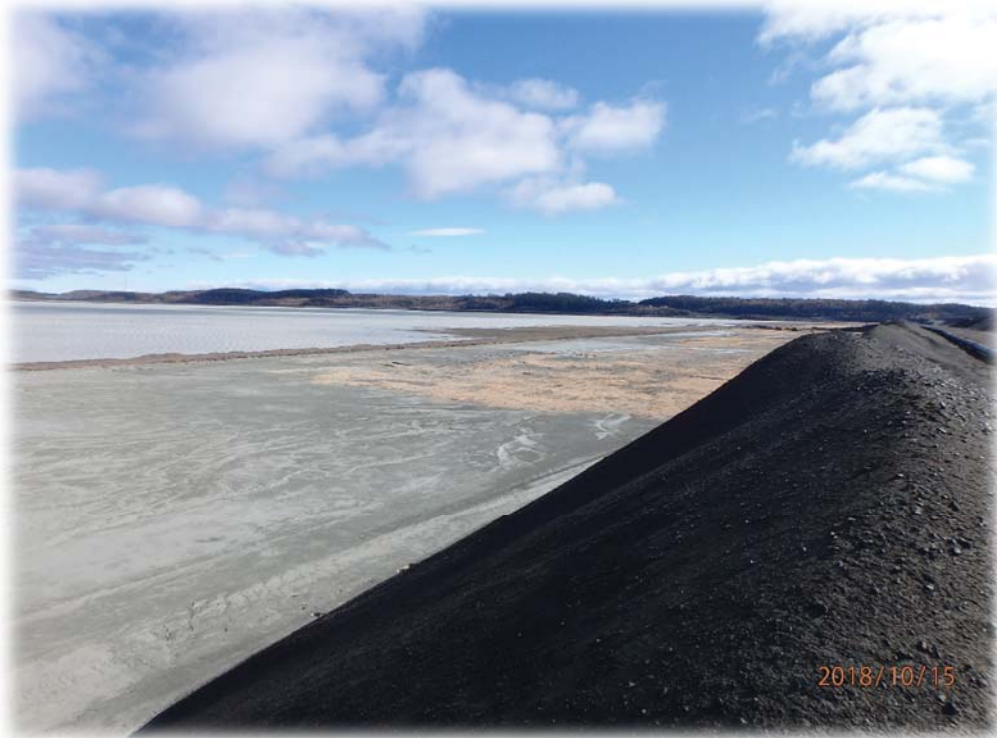
Looking east at area of new super cell beach where fine tailings were recently spigotted
