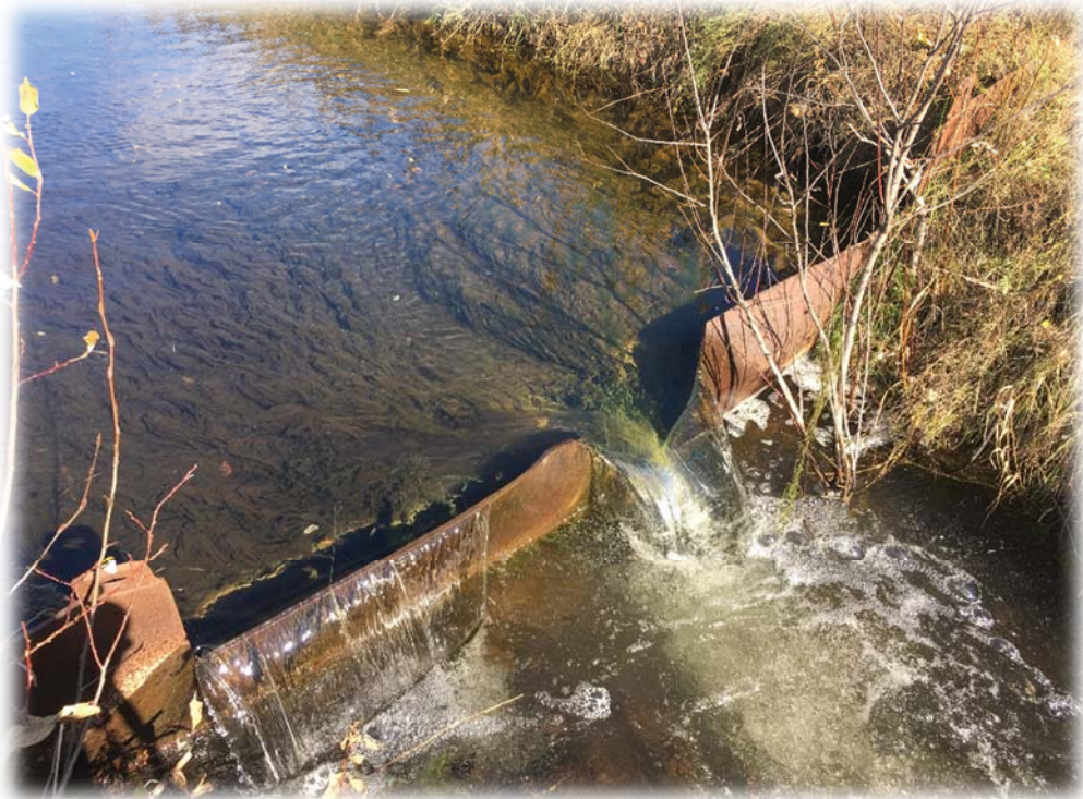
Weir at east end of seepage recovery ditch for main segment of Dam 1
