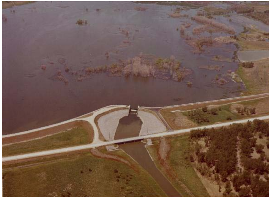
Figure 1-7. Highway 75 Dam on the Minnesota River.
