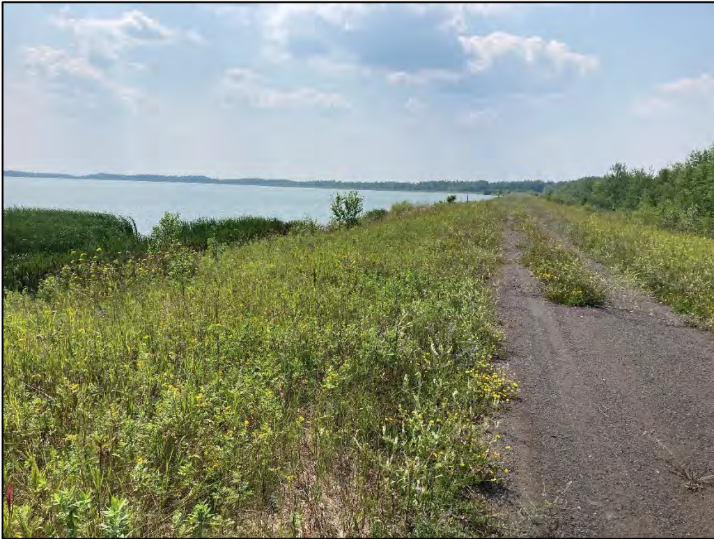
Photograph 55 (IMG_4137): View southwest of the tailings basin berm on August 2, 2021.
