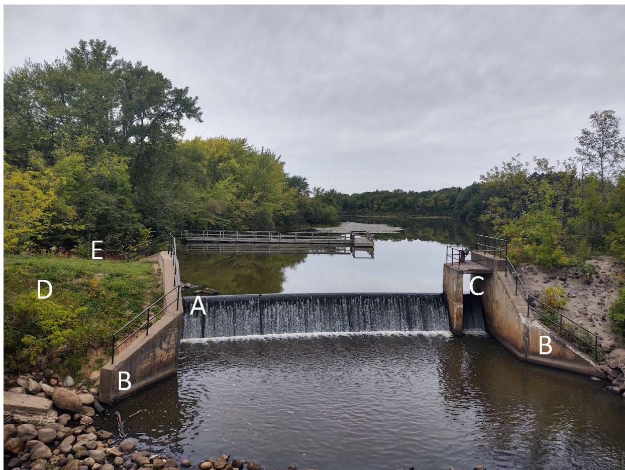
Figure 1-1. Grindstone Dam located on the Grindstone River in Hinckley, Minnesota. The Grindstone River is in the foreground of the picture, the Grindstone Reservoir is located behind the dam. Labels: A. Concrete spillway; B. Left & Right Abutments; C. Sluice gate. ; D. Embankment, and E. Sheetpiling.
