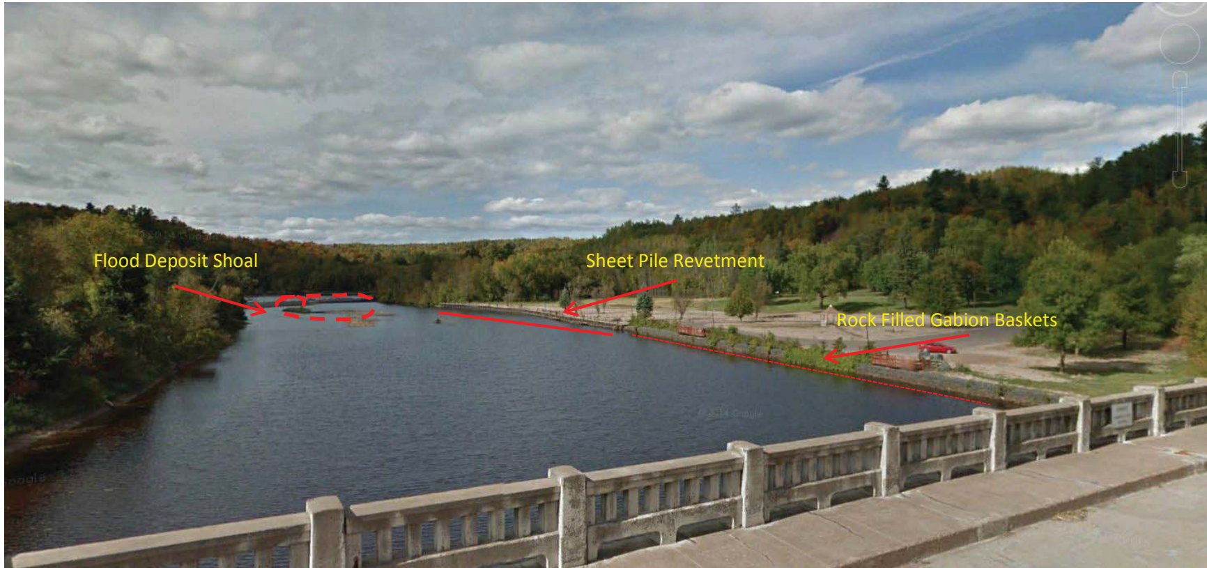
Figure 3: Existing conditions at Chambers' Grove Park showing full extent of the project area with locations of degraded aquatic habitat features identified. View looking west-northwest upstream from MN State Highway 23 bridge at secondary channel, north bank St. Louis River at Fond du Lac.
