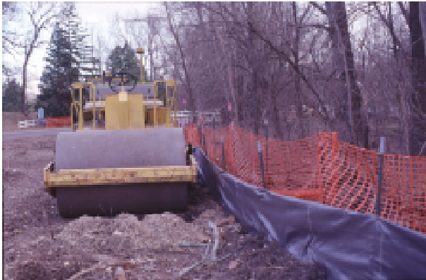
Figure 15. A combination of visual fences and silt fences prevent access to the protected root zone and construction damage to trees as well as runoff.
