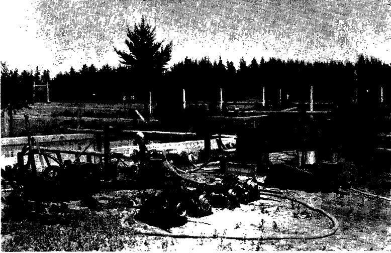
The fire pumps of 1931.
