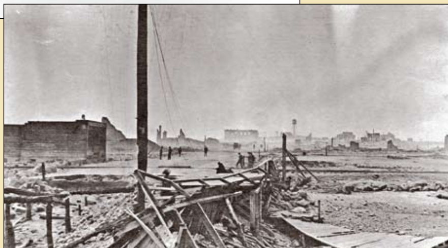
Hinckley after the fire.
