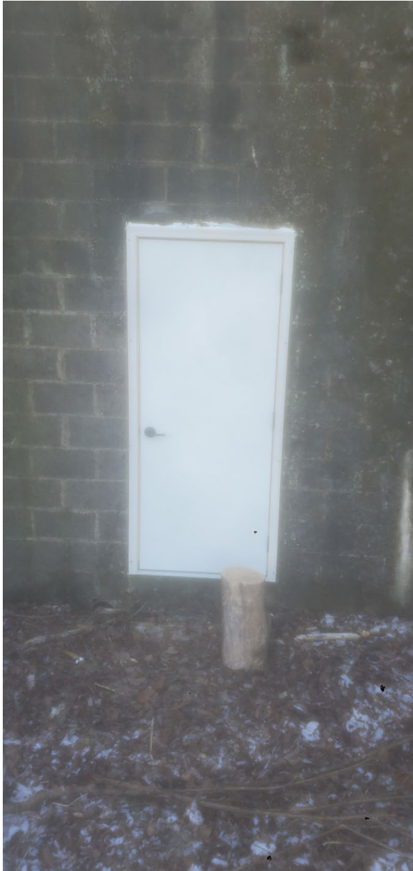
Figure 6. Exterior door for a hibernacula on DNR land. This door was replaced in fall 2024. This door replaced a previous door that began having issues staying securely closed due to weathering. Bats enter this site through a bat portal approximately 5 feet above the door (not included in image).
