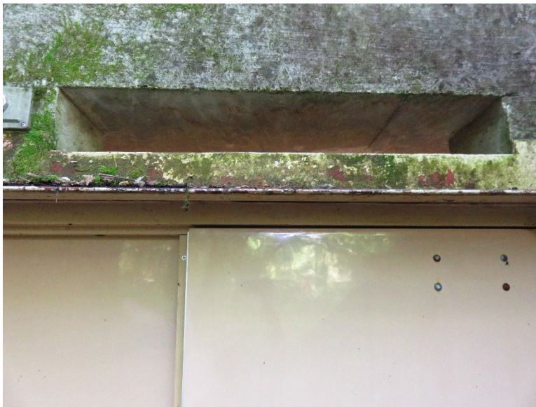
Figure 3. Close up of exterior bat portal entry at the entrance door shown in Figure 2.
