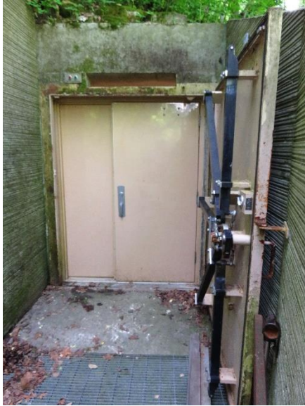
Figure 2. Mystery Cave Entrance 1 Door with exterior barrier open, bat portal visible above door. This entry leads to a cement tunnel that contains a second door to access the cave interior.
