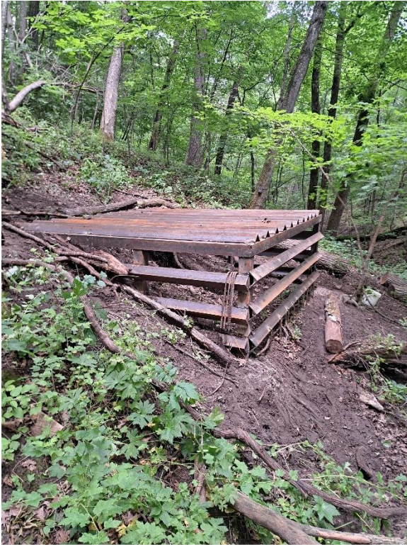
Figure 1. A recently collapsed ceiling in a side passage of Mystery Cave had created a new, unmanaged entrance into the cave. A newly installed 10' x 10' cupola-style bat gate to allow fly-in bat access but block human entry.
