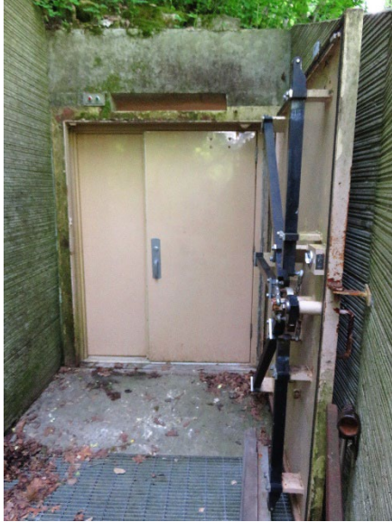
Figure 2. An entrance door to a hibernaculum on DNR land with exterior barrier open, bat portal visible above door. This entry leads to a cement tunnel that contains a second door to access the cave interior.
