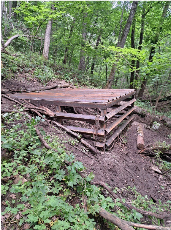
Figure 1. A recently collapsed ceiling in a side passage of a hibernaculum on DNR land had created a new, unmanaged entrance into the cave. A newly installed 10' x 10' cupola-style bat gate to allow fly-in bat access but block human entry.
