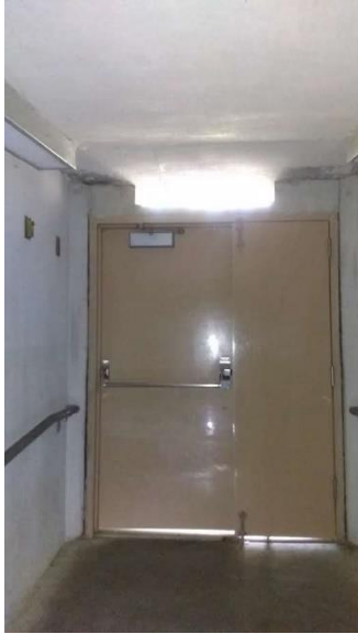
Figure 4. Interior view of outer door at Mystery Cave Entrance 1.
