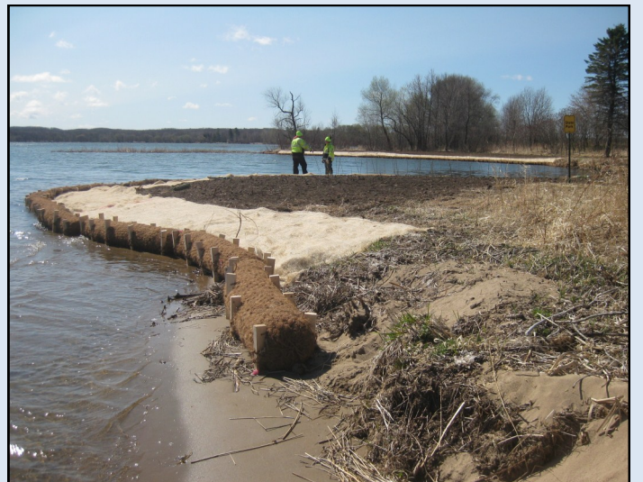
Contractors finish erosion control with willow staking. Willows will take root and help to stabilize the bank. The large log-like roll at the water's edge is called a coconut lag, and is used to accumulate any sediments that do drain off the disturbed soil. Native wetland plants and upland grasses and forbes were seeded in appropriate areas.
