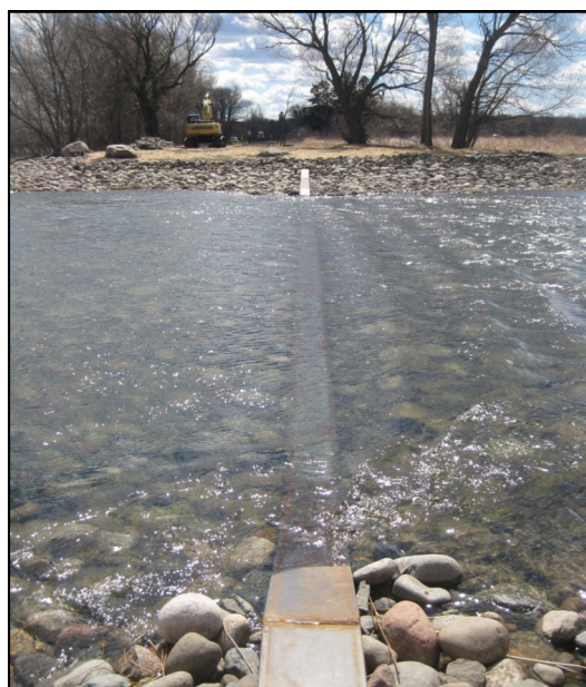
Above two photos: Before and after photos from the mouth of the Rum River. Bottom: Close up of the newly constructed weir dam.
