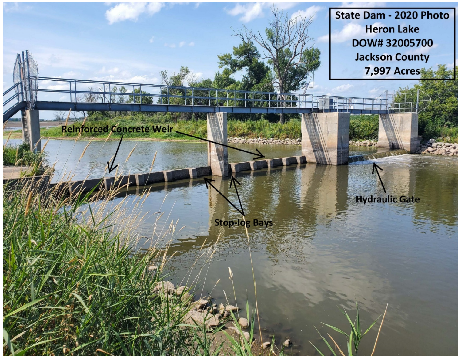
Attachment B. Picture of the State Dam that displays the location of the concrete weir, stop-log bays, and hydraulic gate.
