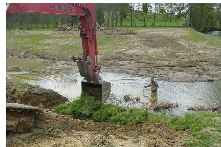
PHOTO: SOD MATTING W/ TOE WOOD APPLICATION
