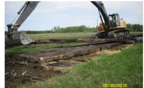
Part F. Removal of the timber mat bridge that was used to span the Ditch Fen area without disturbing the components of the fen that were under the bridge.
