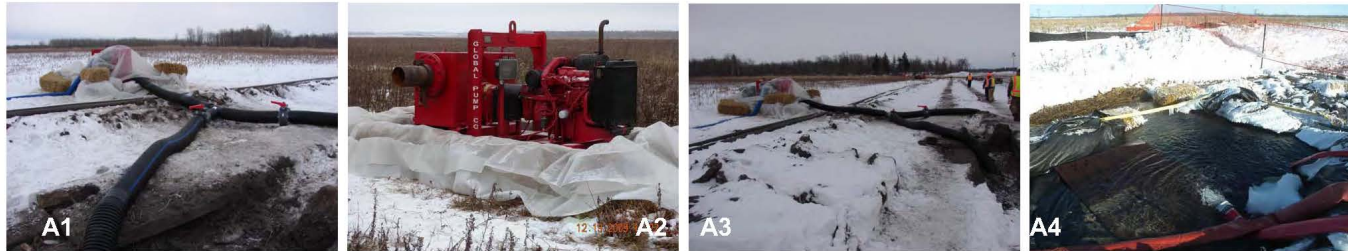
Figure 2.3-3 Drain Tile Installation and Dewatering System
