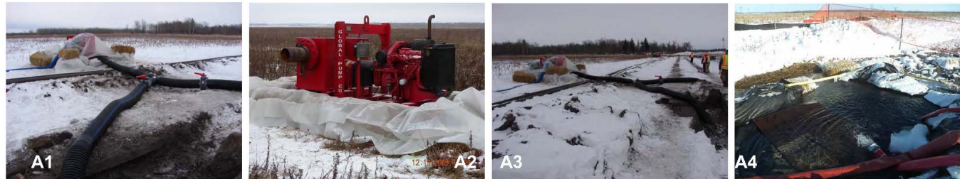
Figure 5.4-1 Drain Tile Installation and Dewatering System
