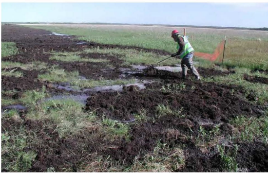
Part D. Restoration staff continuing to spread a thin layer of local peat topsoil in areas where the sod has subsided to below pre-construction contours.
