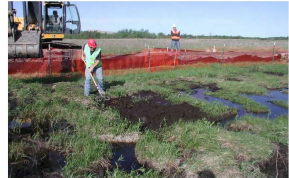
Part C. Because some of the sod pieces had subsided below the pre-construction contour and were very fragile because they were covered with water, a thin layer of peat was used to raise the ground surface elevation. Plants are expected to grow through the thin peat layer.
