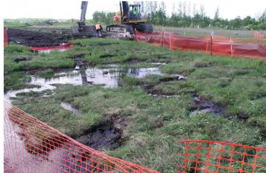
Part B. The sod portion of the Ditch Fen area after the pieces of sod that were above the pre-construction grade had been pressed down to the pre-construction level.
