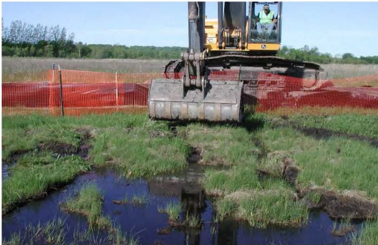
Part A. Because some sections of the sod replaced in January were above the pre-construction elevation, a long-stick backhoe with an 8-foot wide bucket operating off of the timber mats was used to gently press the sod down to the pre-construction elevation.
