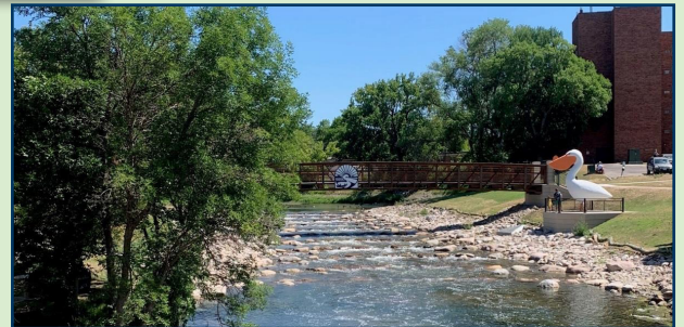
The deteriorating dam in Pelican Rapids, MN was modified into a Rock Arch Rapids winter 2022/2023. The ramp gradually steps down the water 5 feet over 12 arches.
