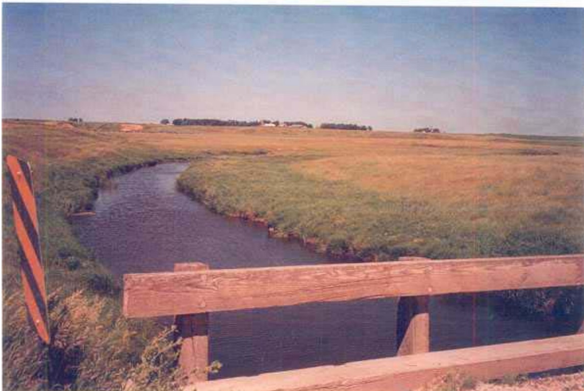
Figure 28. (top) Gravel mining at site immediately adjacent to Telemetered turtles, including three adults, BBW, BBP, and BBCI, frequented the and streambanks on either side of the bridge on (bottom) Another gravel operation was active on the west side of of Rock River; gravel piles are visible in upper left horizon, looking WSW
