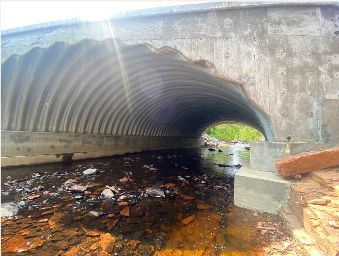
Photo: Fish and wildlife friendly and climate-adapted road crossing, Hockamin Creek, Jeff Jasperson, Minnesota Pollution Control Agency
