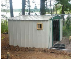
Free standing structure
