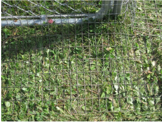
Protection from burrowing predators (wire mesh forms an L)
