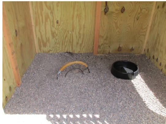
Pea gravel for flooring (easy clean-up—rake out/spray out waste)
