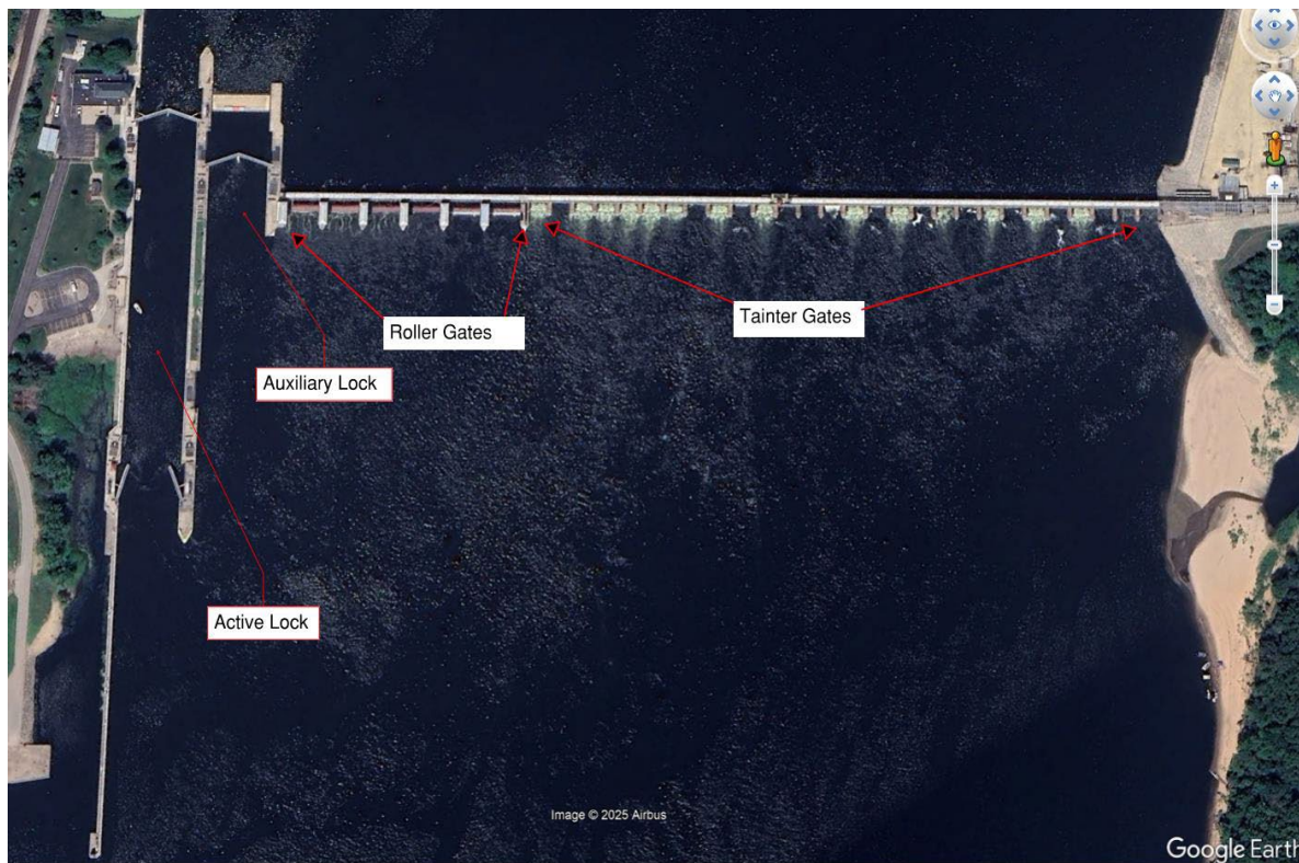
FIGURE 1.3.4-1. Overhead View of LD5
