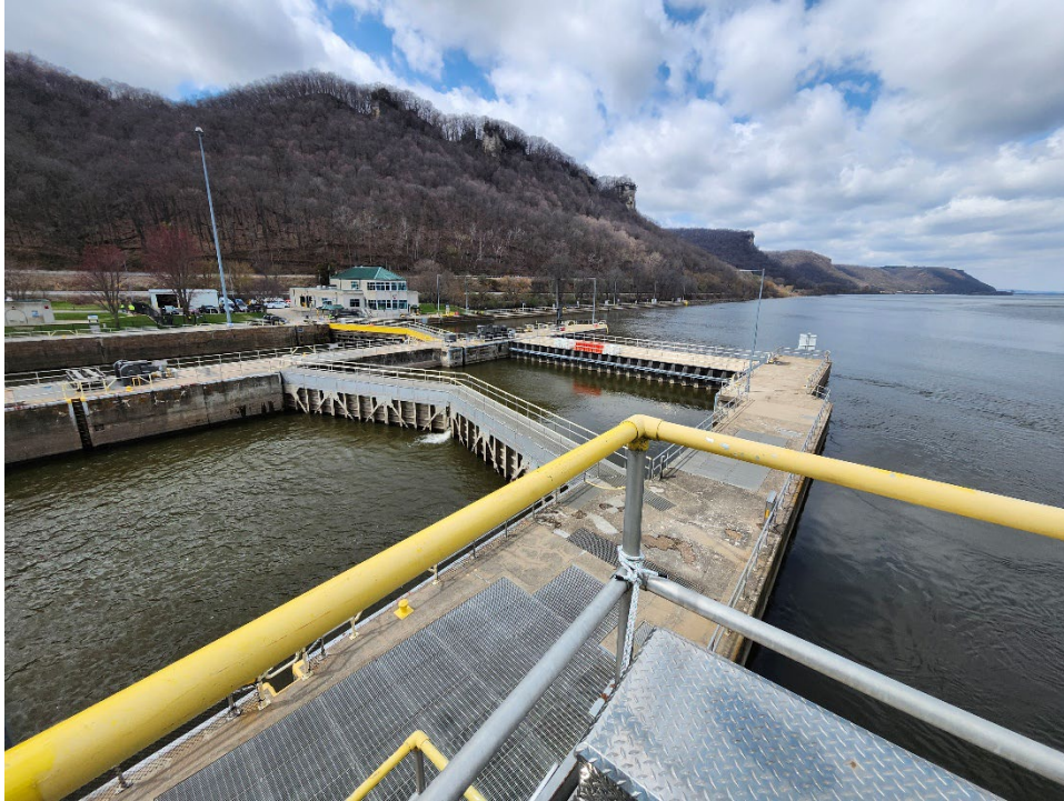
FIGURE 1.3.4-3. Upstream End of Auxiliary Lock (Primary Lock is to the left and above of the auxiliary lock in the image)
