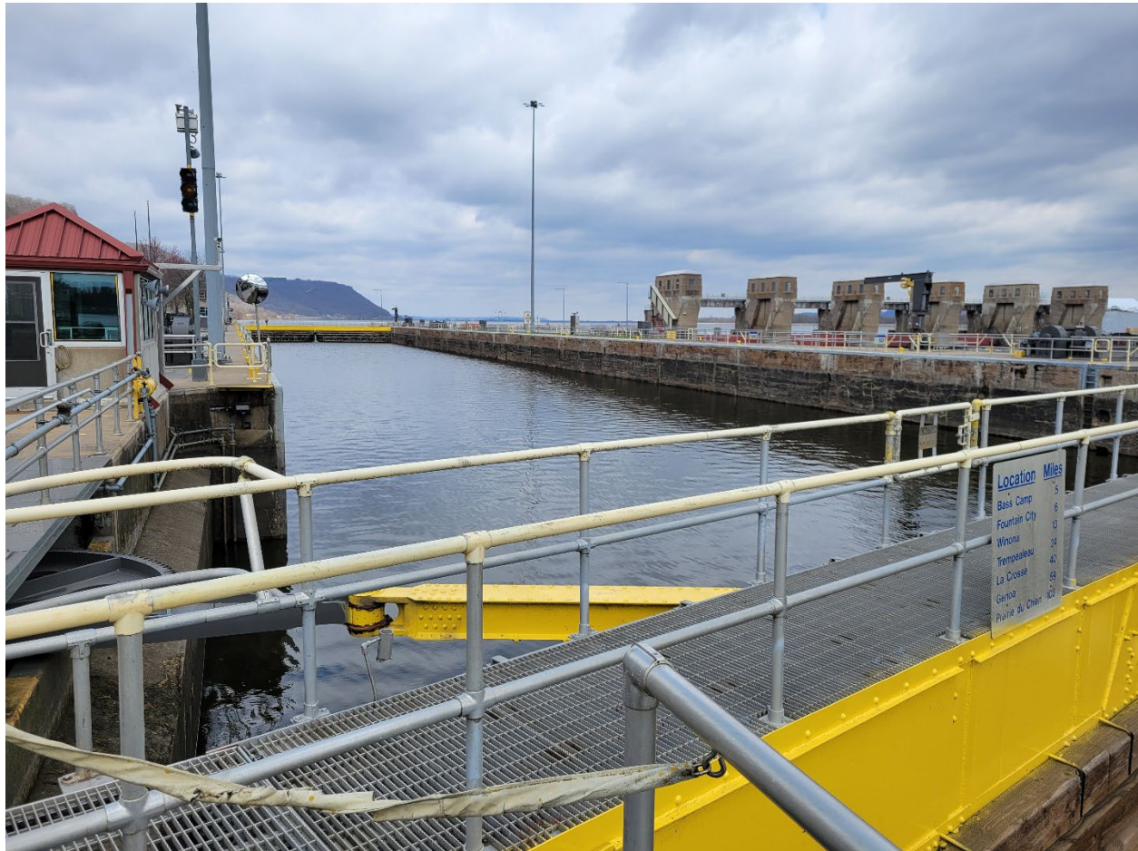
FIGURE 1.3.4-2. Photo of main lock taken from miter gate looking upstream to north end of main lock
