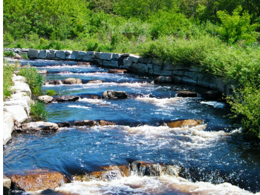
FIGURE 2.6-1 Rock Ramp Fishway
