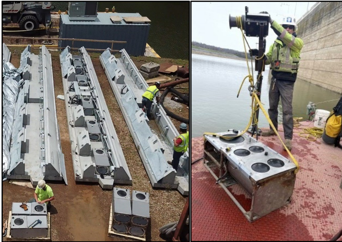
Figure 6-10. BAFF SPA at installation and after repair. (Left) BAFF Installation Lake Barkley (Photo credit: Kentucky Department of Fish and Wildlife Resources, Used by Permission, https://www.fws.gov/media/baff-installation-lake-barkley ). (Right) The projector design changed to include a 5 “window” interface. Accessed 2025 DEC 07; https://www.mainstreamdivers.com/MoranSharedCmsContent/CaseStudyView.asp?NewsID=79 )
