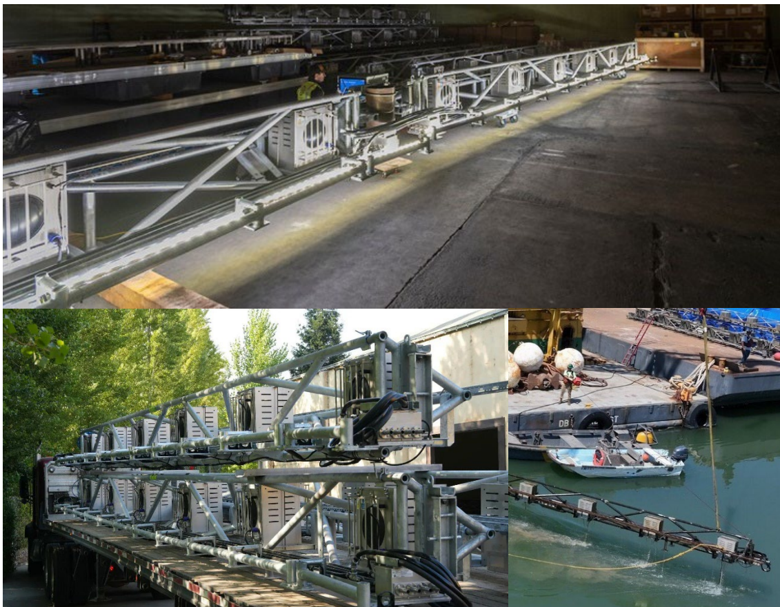
Figure 6-5. Installation of the BAFF at Georgiana Slough, CA. (Top) BAFF Testing for Georgian Slough in Hood, CA ( water.ca.gov/News/Blog/2023/Sep-23/DWR-Installs-Illuminated-Bubble-Barrier-to-Help-Young-Salmon-Migrate-Safely-Through-Delta ). (Left) BAFF Components before installation at Georgiana Slough. (Photo credit: Fish Guidance Systems, LTD). (Right) Seasonal removal of the BAFF at Georgiana Slough (Photo credit: California Dept. of Water Resources; Accessed on 07 DEC 2025 https://x.com/CA_DWR/status/1930705561542066274 ).
