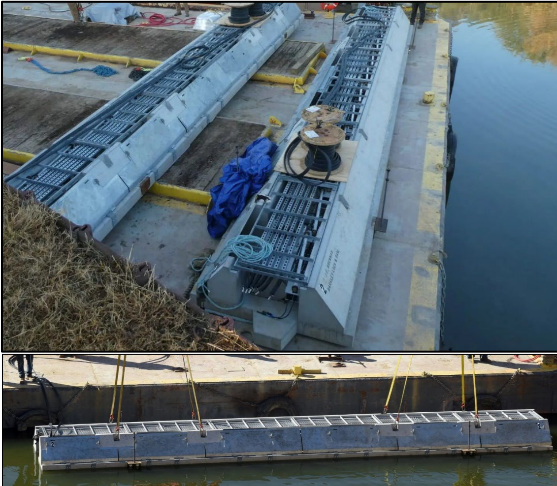
Figure 6-8. Installation of the BAFF at Barkley Lock and Dam, KY. Installation of the BAFF at Barkley Dam (Top Photo Credit: Accessed 2025 DEC 07; https://fgs.world/invasive-carp/ ; Bottom Photo Credit: Leon Roberts, USACE).
