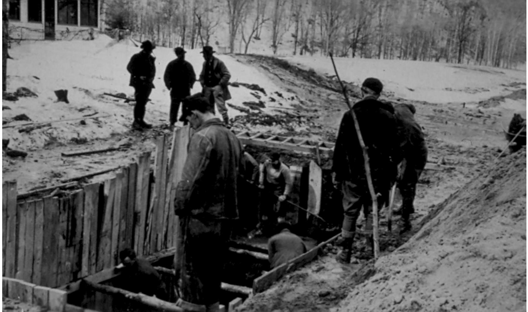
When you flush a toilet in the North Picnic Grounds, you are utilizing the original septic system constructed by the CCC boys in the winter of 1935. The fact that this system still functions over 80 years later is a testament to its design.
