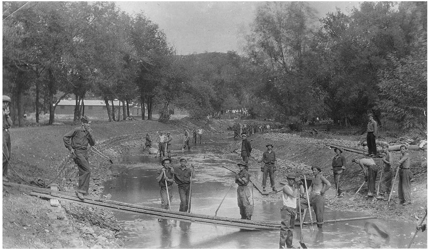
Much of the quarried stone was used as rip-rap along the river. This common practice helped prevent streambank erosion.
