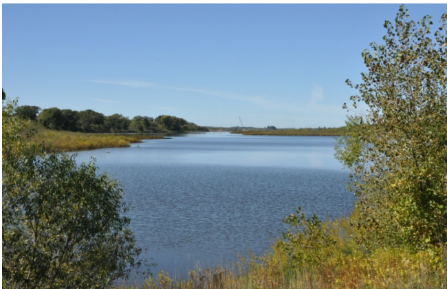
The Project built two small dams and dredged the bottom of the “Watson Sag,” shown here, so high water from the Chippewa River would flow into Lac qui Parle Lake rather than flooding Montevideo and other cities.
