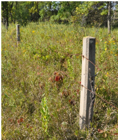
WPA workers made concrete fence posts which they installed in a 3-mile line along the southwest boundary of the Flood Control Project. The posts can be seen on the west side of LQP County Road 33 near the LQP State Park Lower Campground.
