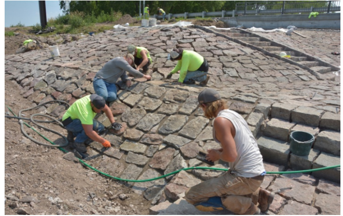
Restoring the stonework at the Milan Bridge in 2021.
