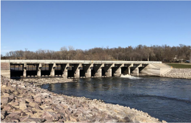
Lac qui Parle Dam, completed in 1941.
