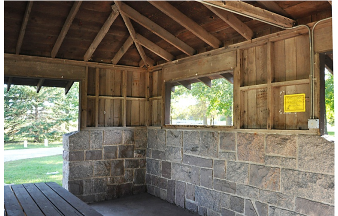
Stone and timber picnic shelter at Watson State Scenic Wayside (now Watson Lions Park), completed in 1939.
