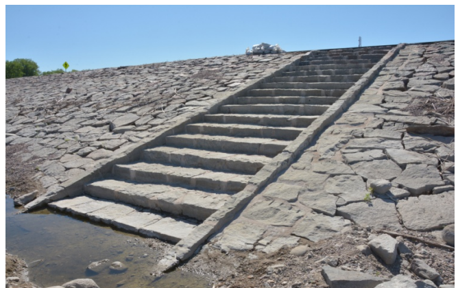
Stone staircase on the causeway just west of the Milan Bridge. The WPA built the staircase around 1939. It was restored in 2021.
