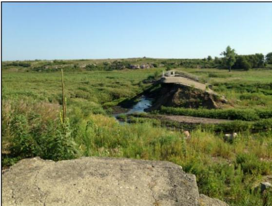
Emergency Spillway washed out after flood.
