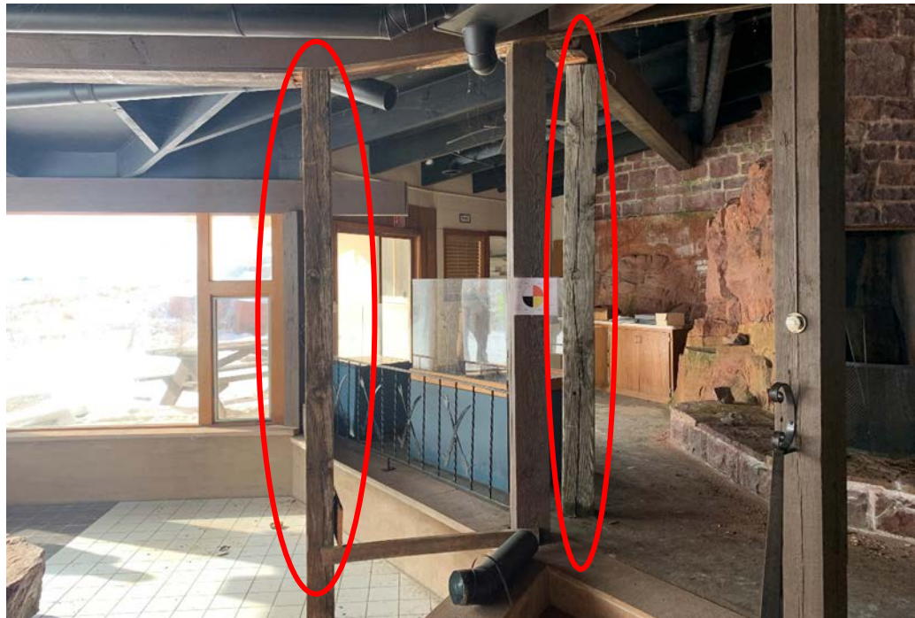
Photo 19 Shoring to support beams rotting at bearing. The un-circled posts are original construction
