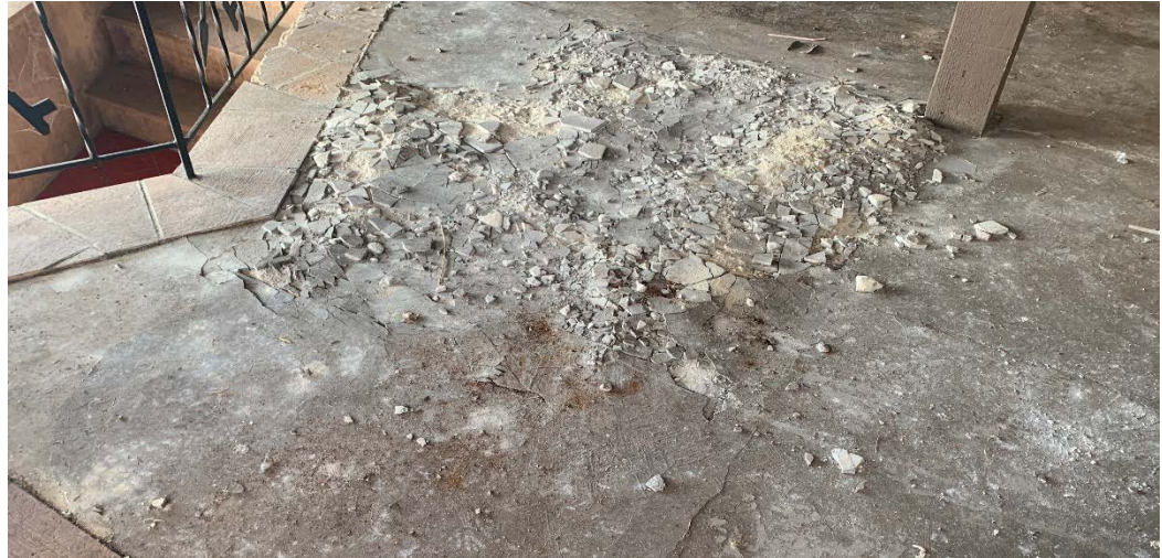
Photo 22 Failing interior concrete slab
