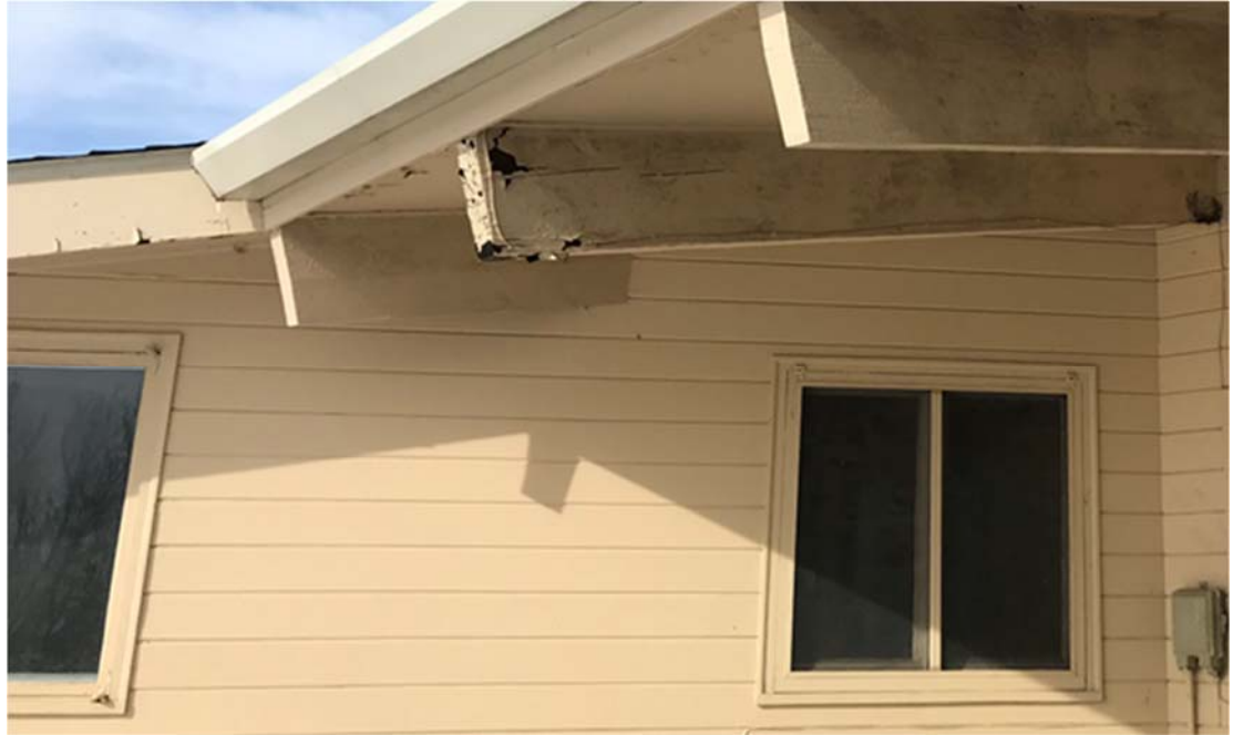
Photo 20 Rotting roof beam at building exterior
