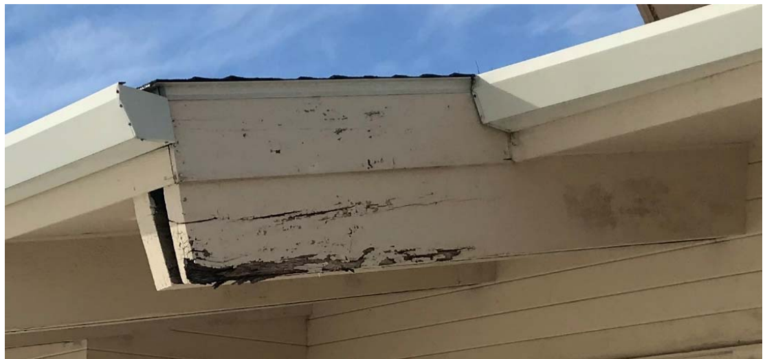
Photo 21 Rotting roof beam at building exterior
