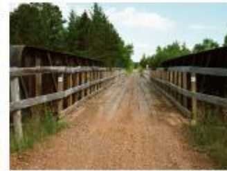
If a summer-use bridge is used for a snowmobile trail, the surface of the trail and deck should be smooth and flush. The deck boards should have minimal gaps to hold snow. Railings are also required.
