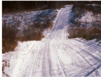
Approaching hills at a right angle is important with snowmobile trails to prevent rollovers. On steep slopes on two-way trails, separating the uphill and downhill sections is sometimes used to increase safety and reduce the potential for conflict. With the open sightlines and modest grade of this hill, two-way traffic on a single 12- to 14-foot tread works well.
