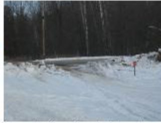
A narrow tread caused by snowbanks poses two concerns: 1) it reduces the sightlines from the trail and roadway and 2) it squeezes riders into a single path just when they are about to make a crossing. On designated trails, avoid this whenever possible.
