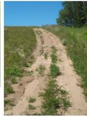
Even seemingly stable soil conditions can be susceptible to erosion when a snowmobile trail corridor becomes a de facto ATV trail. The key point is that all trails must be designed for their purpose. It should never be assumed that a trail corridor for one purpose will be suitable for another until it is assessed for that purpose.
