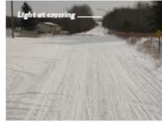
Along with proper signage, a light is added at this trail crossing to improve safety. The flatness and straightness of the road conversion reduced the visual cues associated with identifying this intersection, warranting the addition of the light.
