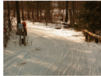
Provide adequate visual cues of an approaching tight curve to enhance trail safety. From this direction, the gate and other signs at the trailhead alert the rider of the approaching curve. From the other direction, a warning sign is provided about 100 feet prior to the curve to alert riders to slow down and approach with caution.
