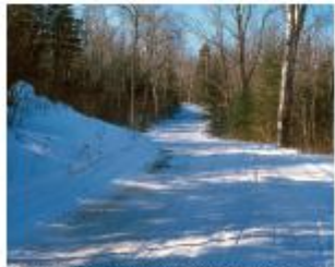
Longer, flowing curves with adequate sightlines are preferred for snowmobile trails. Sightlines should be long enough for the rider to react to oncoming conditions but not so long as to entice excessive speeds.
