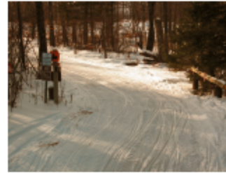
Provide adequate visual cues of an approaching right curve to enhance trail safety. From this direction, the gate and other signs at the trailhead alert the rider of the approaching curve. From the other direction, a warning sign is provided about 100 feet prior to the curve to alert riders to slow down and approach with caution.
