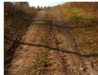
The lack of ground cover on this steeper hill is allowing erosion to take hold, making the trail unsustainable for summer use and increasingly rough for winter use.
