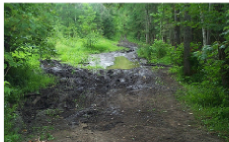
This otherwise sustainable snowmobile corridor is not well suited to summer ATV use, as the photo clearly illustrates. An ongoing occurrence of this type of impact only leads to more restrict uses, sometimes even for those the trail was designed to accommodate.
