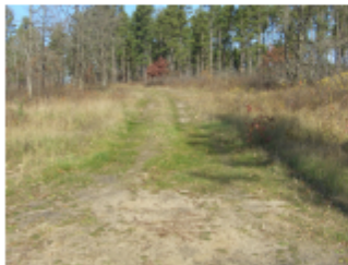
A level, grass-surfaced corridor is optimal for snowmobile trails. Mowing the trail just before the season can reduce the amount of snow needed to create a usable base.
