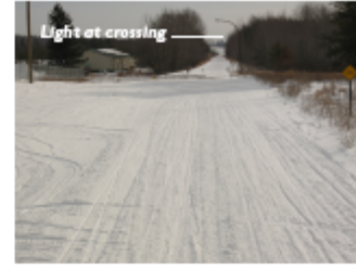
Along with proper signage, a light is added at this trail crossing to improve safety. The flatness and straightness of this rol conversion reduced the visual cues associated with identifying this intersection, warranting the addition of the light.
