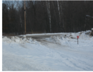
A narrow tread caused by snowblowers poses two concerns: 1) it reduces the sightlines from the trail and roadway and 2) it squeezes riders into a single path just when they are about to make a crossing. On designated trails, avoid this whenever possible.
