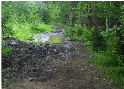
ise sustainable snowmobile corridor is not well suited to summe the photo clearly illustrates. An ongoing occurrence of this type nly leads to more restrict uses, sometimes even for those the signed to accommodate.
