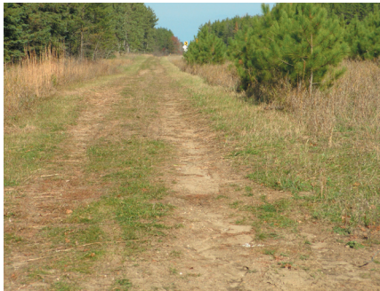
This even and smooth grade with vegetation and a slight cross-slope is ideal for a snowmobile trail.
