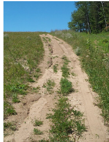
Even seemingly stable soil conditions can be susceptible to erosion when a snowmobile trail corridor becomes a de facto ATV trail. The key point is that all trails must be designed for their purpose. It should never be assumed that a trail corridor for one purpose will be suitable for another until it is assessed for that purpose.
