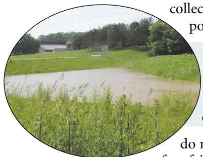
Urban stormwater detention ponds store excess runoff.
