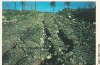
Properly placed culvert above drains road well and water runs clear. Culvert on right provides poor drainage and degrades water quality.
