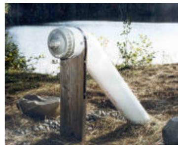
*Typical dry hydrant installation.*
