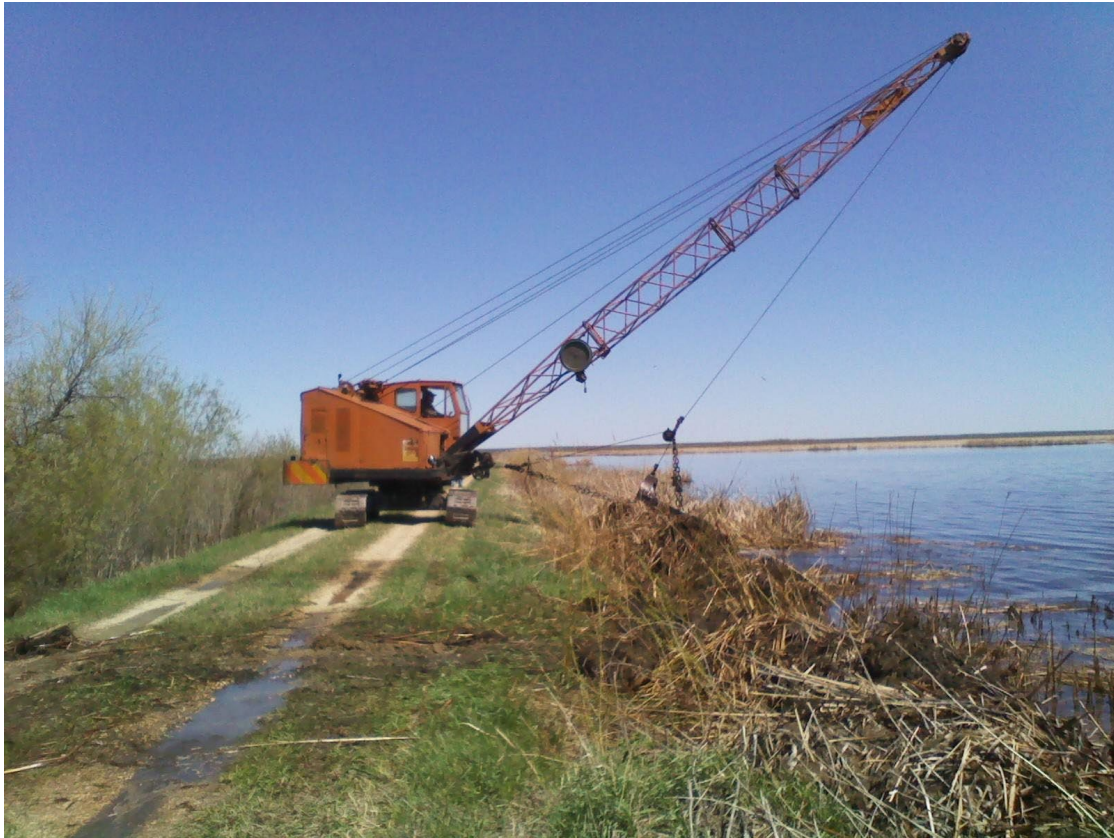
7 Figure 43. Photo of the dragline excavator removing cattails
