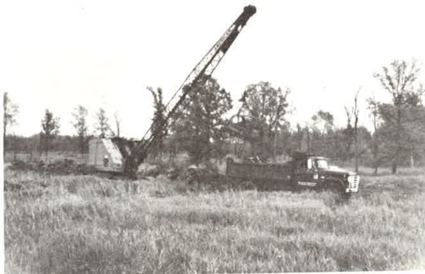
A dragline is used to construct potholes for waterfowl.
