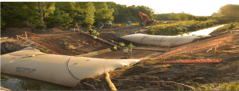
Giant bladders divert Mayhew Creek around the electric barrier construction site.
