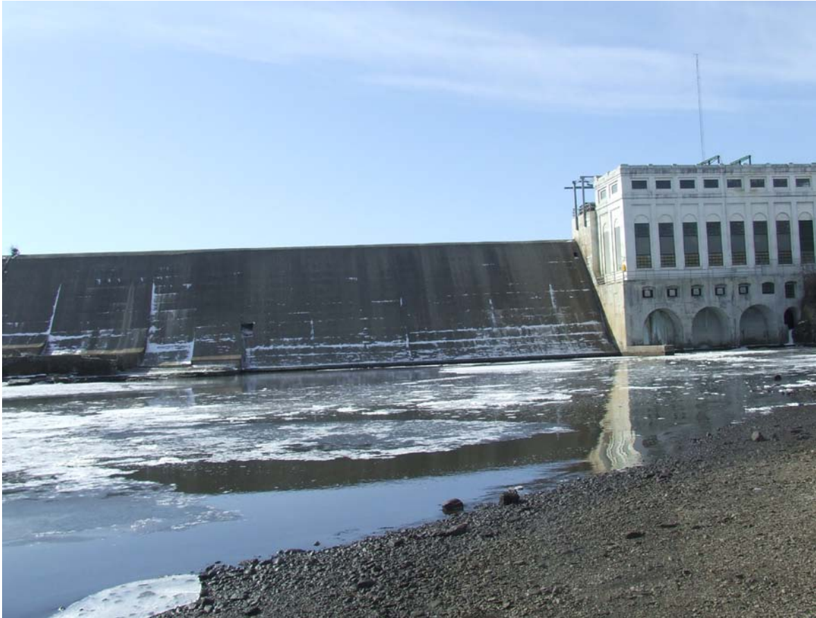
Figure 2. Zumbro Dam March 2009.
