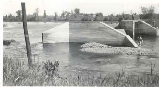
View looking north. Note marking of dyke section on back of end wall before failure.
