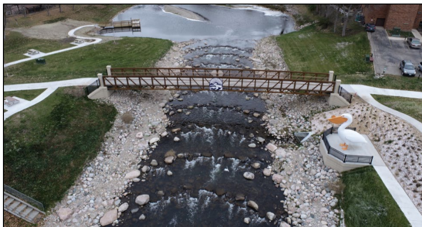
Example of a rock arch rapids design used at Pelican Rapids after removing the existing dam.
