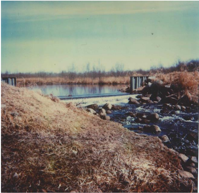
Minnewawa Creek Dam at Lake Minnewawa. While not very high, it still prevents fish from moving back up into the lake. This is especially true of smaller juvenile fish when water levels are low.
