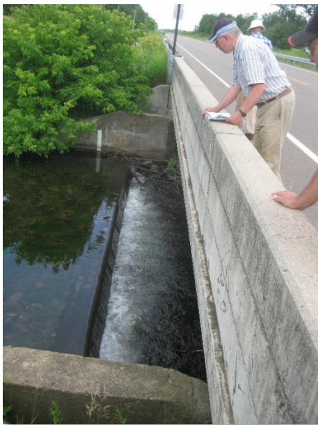
Another example of a low head dam that prevents fish movement on the Ripple River. This is at the outlet of the Ripple River at Spirit Lake. Here, the main issue is with juvenile fish. There is a spawning area just below the dam and while adult can usually make it back up into the lake, later in summer the juvenile walleye cannot navigate the barrier. Members of the Aitkin County Water Planning Task force toured the site a few years ago.
