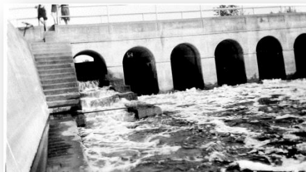
US Army Corps of Engineers Dam, at outlet of Big Sandy Lake near Libby. Note the "fish ladder" just right of the stairs. While this type of fish passage may have worked for salmon, it would not work for most fish in Big Sandy Lake. The only time fish can swim back up into Big Sandy is when the Mississippi River and Big Sandy are about the same elevation. Most recently this occurred during the flood of 2012.
